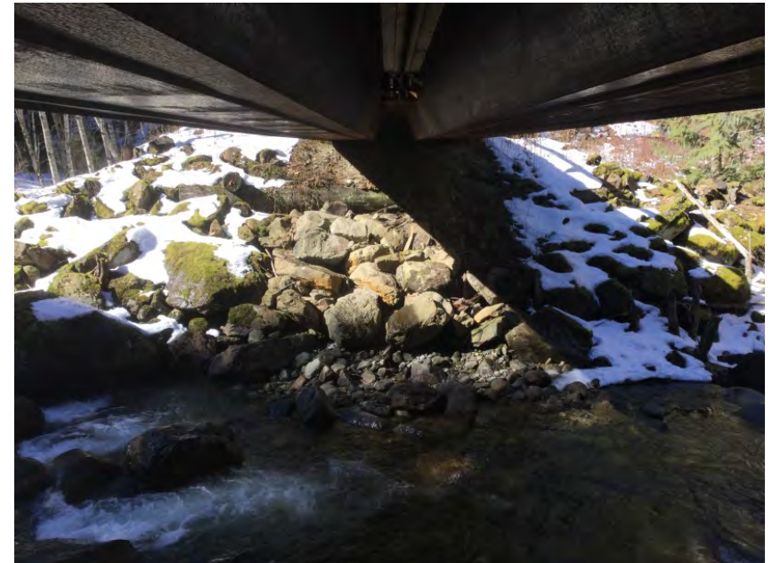
Left Bank Abutment when facing downstream
