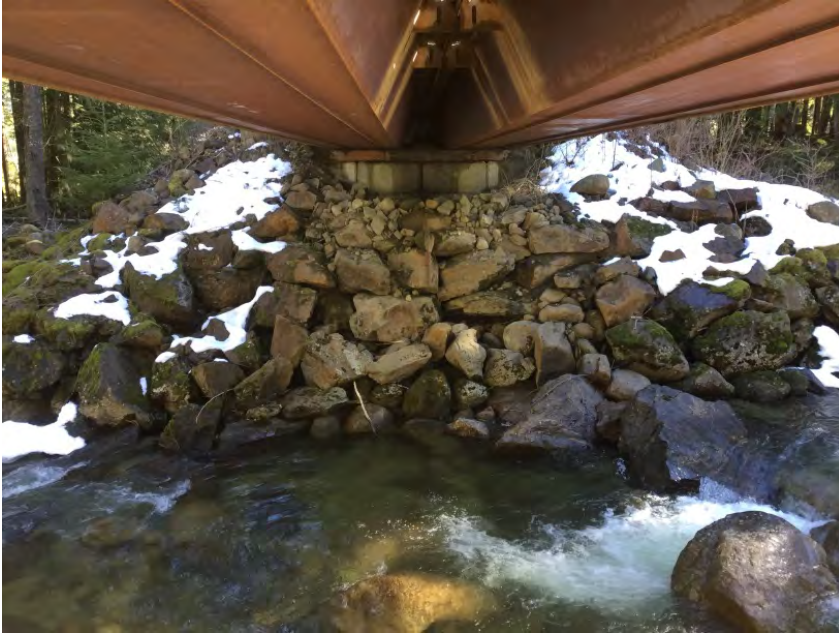
Right Bank Abutment when facing downstream
